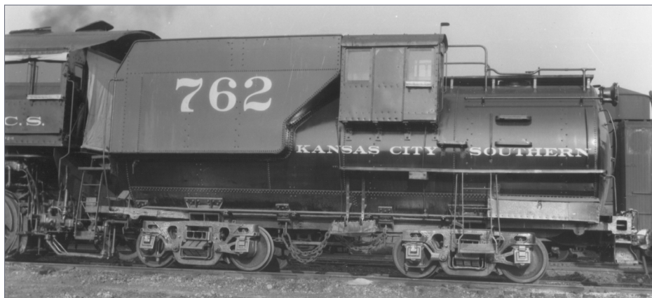
27. The KCS short fat Vanderbilt tender for the G1 class articulated. Harold Vollrath photograph from the collection of Dr. Nicholas Muff
