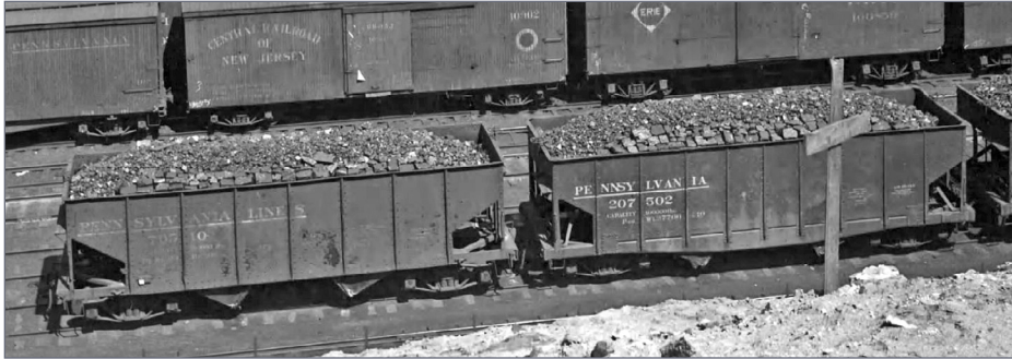
16. Cleveland, Ohio, circa 1910. Shown here are GLA (left) and GL (right) cars. All the freight cars in this photo appear to be riding on arch bar trucks. Note the GLA is lettered for PENNSYLVANIA LINES and the GL is lettered as PENNSYLVANIA. Also note the coal is not uniform and is randomly sized. I love those wood-roofed boxcars behind the hoppers.
