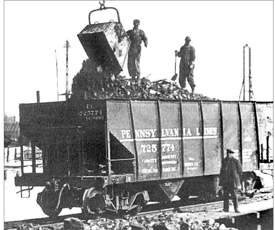
18. In a 1916 image, a three-man crew loads Pennsylvania Lines 725774 one bucket at a time. Note the P.L. reporting marks on the car end. Photo from Railway Age Magazine
