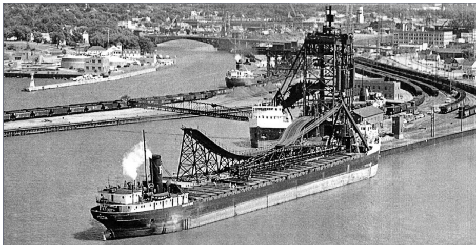
41. Looking south from Lake Erie, this view shows it all. The modern B&O coal dock in the foreground began operation in 1948 – the year your author was born. Behind it stands the ore unloader that replaced the Brown Hoists about 1920. The coal and ore docks each had their own pier jutting into Lake Erie. ohiowea.org
