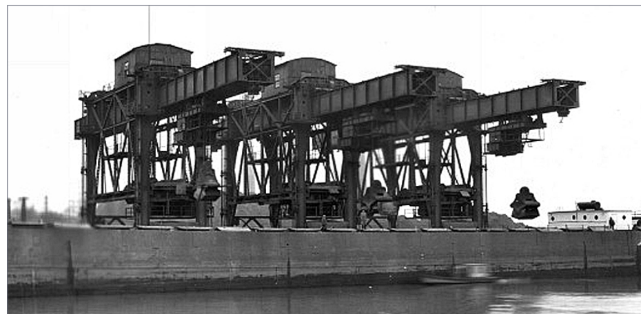
39. Closeup of the Lorain ore unloaders, installed in Lorain about 1920. They were designed between the time of the Brown Hoists and the Hulett ore unloaders. No Hulett unloaders ever got used in Lorain. The above unloaders worked well, and lasted until the 1970s, some fifty-plus years of hard service. Great Lakes Collection, BGSU
