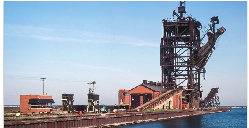
42. Here is the larger McMyler coal dumper that replaced the old No. 2 dumper in 1948. It sat at the very end of the harbor on the west side of the Black River. I believe it was demolished about 1980. Beyond this pier you can see Lake Erie. photographer unknown, Jim Six collection
