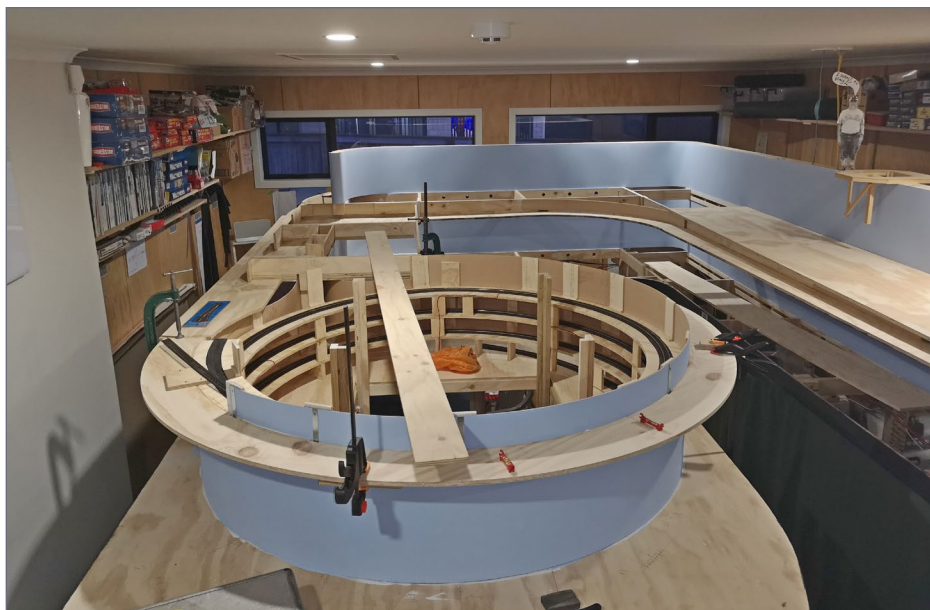
17. Helix run around and connection from east and west.
