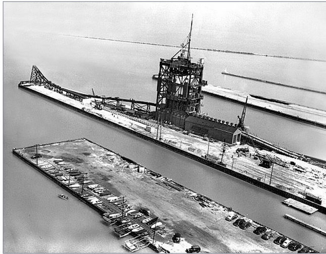
40. This 1947 photo shows B&O No. 3 coal dumper a few months before being placed into service. This was one of the last and most modern McMyler coal dumpers on the Great Lakes. Great Lakes Collection, BGSU
