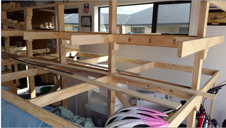
6. Joining the tree frames together.
