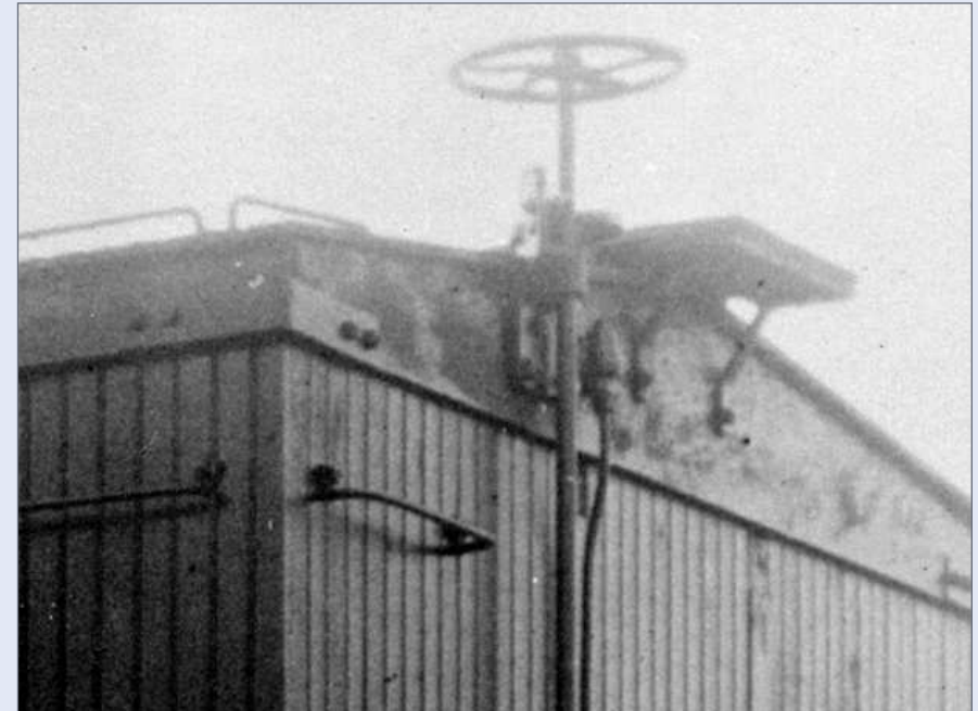
2. The enlargement of the hand brake mechanism in the builder's photo doesn't help much but it's obviously different than the standard brake ratchet and pawl.
