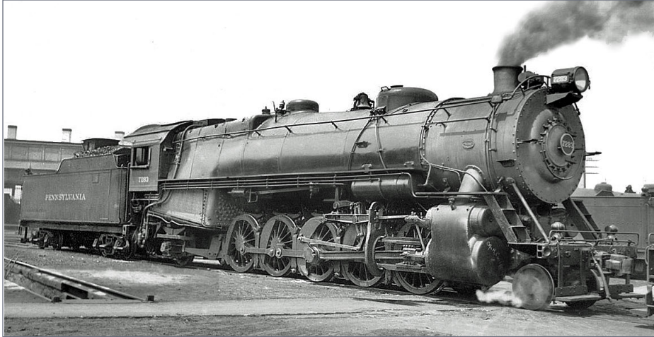
13. PRR N2sa 7283 at Urbana, Ohio in 1942. The tender sports a doghouse but has no coal bunker extension, and the lettering on the side is of the condensed script applied until 1946. Ray Breyer collection
