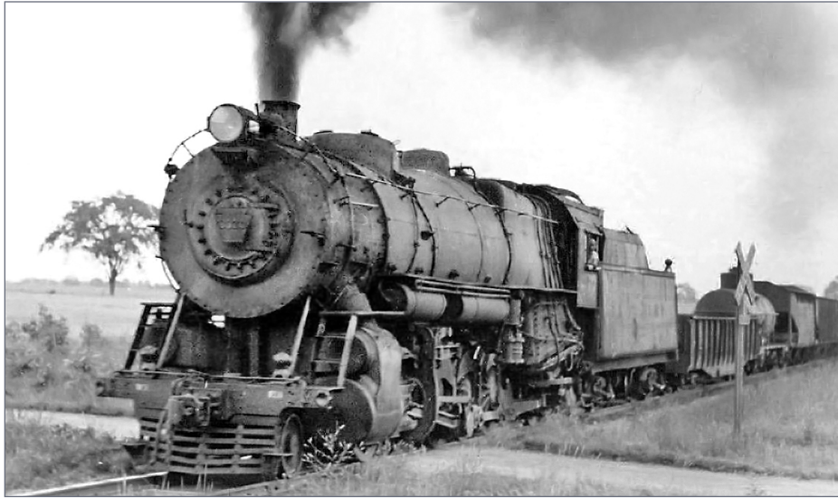
16. This photo shows an unusually configured N2sa locomotive leading a long southbound freight near Vicksburg, Michigan in 1948. The locomotive features a keystone shield centered on the smokebox front, and a cowcatcher type pilot, both more commonly associated with passenger locomotives. Ray Breyer collection
