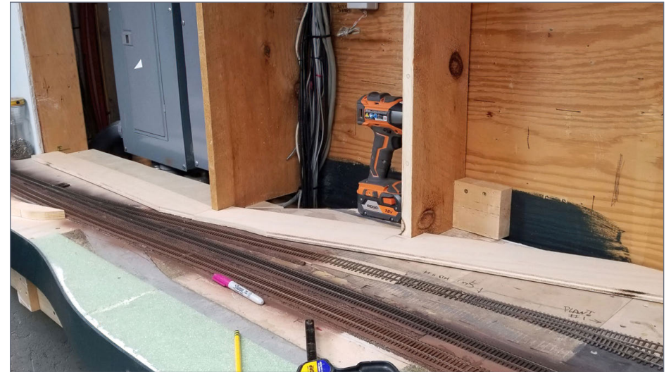
6. I cut horizontal plywood guides for the backdrop and test-fit them to make sure they followed the contours of the wall.
