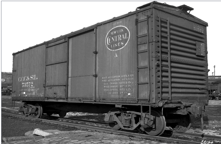
8. C.C.C.&St.L. 53572 was a 36' 3" fish belly boxcar with 80,000-pound capacity.
