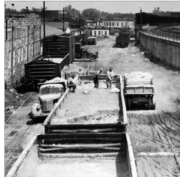
28. Here a tank car of road asphalt has been spotted on the East Shumala team track, to be unloaded by workmen from Guadalupe Paving.
