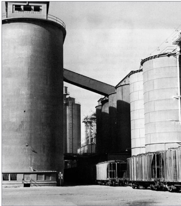
11. This photo from the mid-1950s shows covered hoppers spotted for loading at Southwestern Portland Cement in Victorville, California. The storage silos dwarf the 70-ton hoppers. Don Sims, photo
