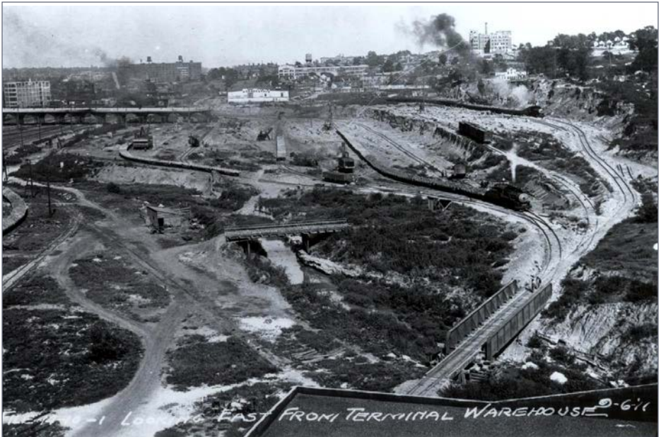
11. Early site preparation. OK Creek can be seen meandering from upper-left to lower-right.
