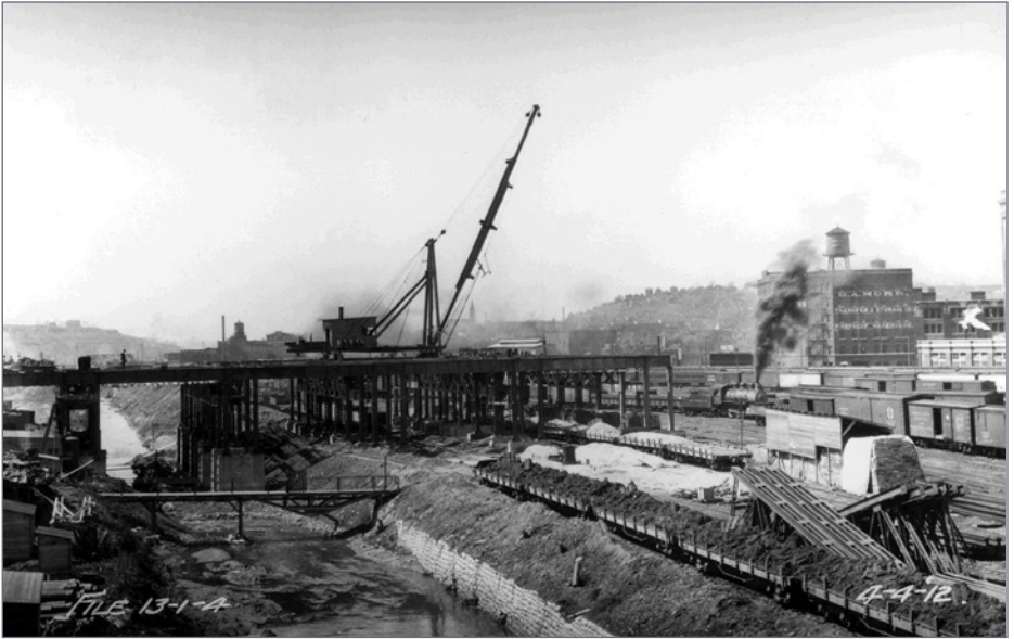
12. Placing support columns for the waiting room.
